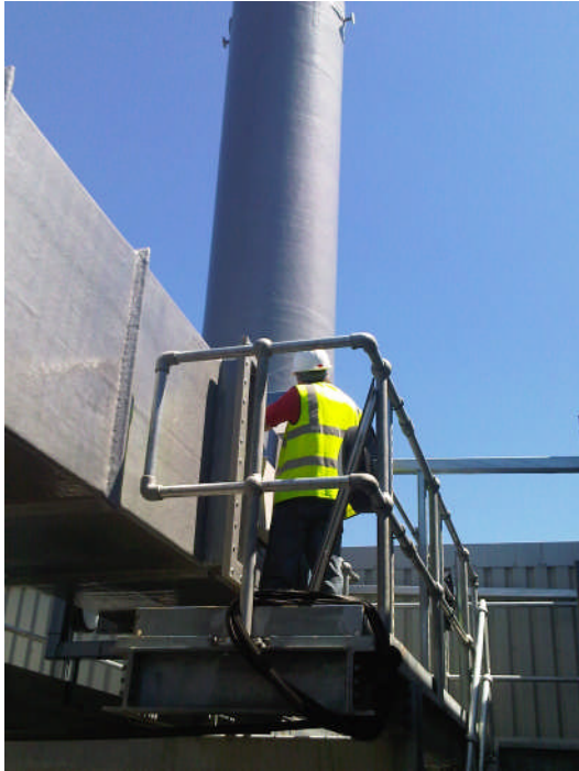
Berthold engineer installing a stack monitor at a PET facility
