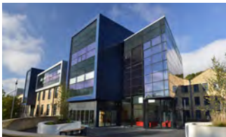
Neutron R&D Centre Huddersfield UK
