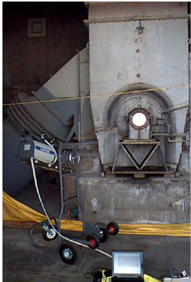
Figure 5-1. In situ measurement of Fan No. 3
