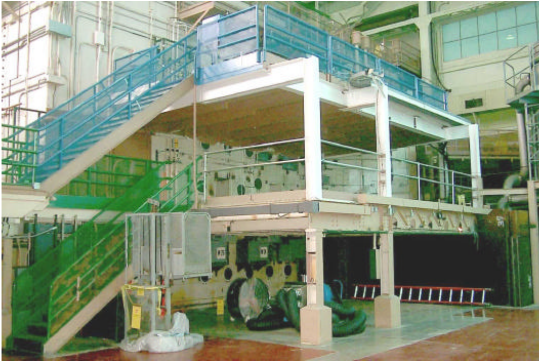
Figure 5-2. West face of the BGRR showing access to experimental port locations
