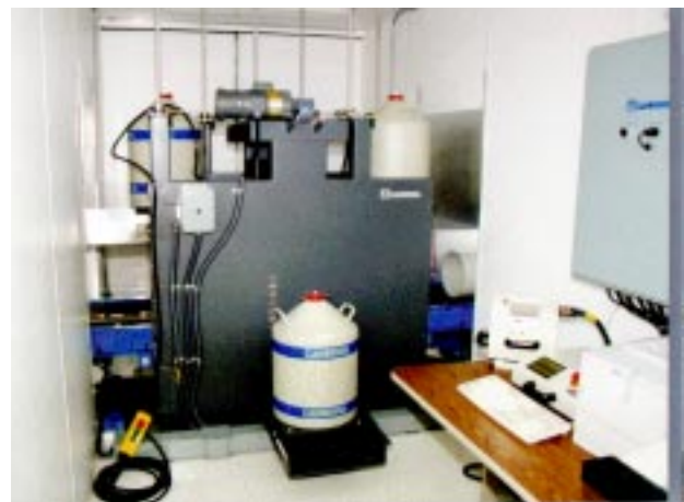
Figure 3. Interior of Unit
